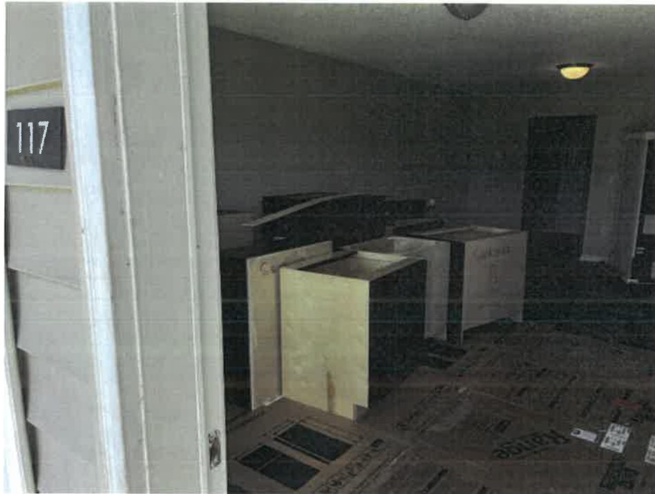
Building J- cabinet delivery
