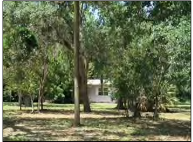
VIEW OF EXISTING IMPROVEMENTS
